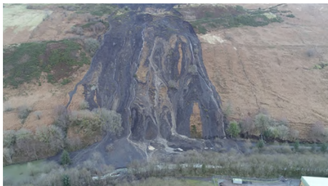
Tylorstown Landslip ( rctcbc.gov.uk )
